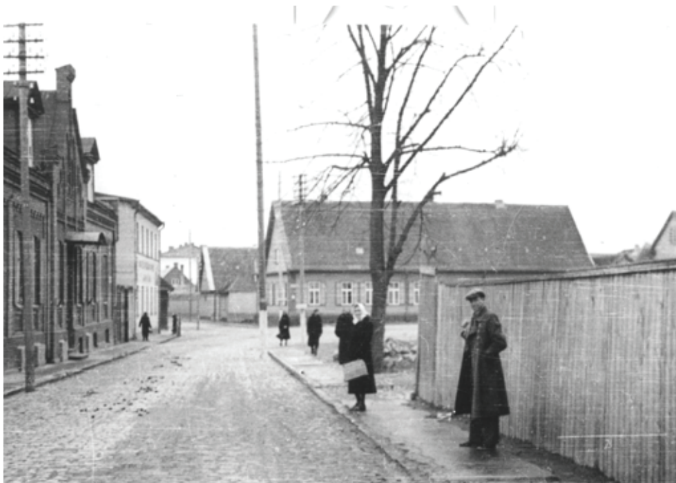
Fig. 11. The intersection of Vecpilsētas and Dobeles streets at the Western Gate, the 1930s. Source: History and Art Museum
